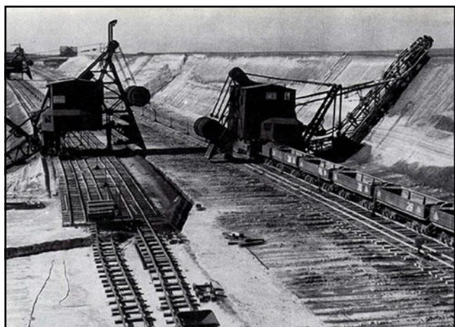
Overburden stripping at the Palmnicken mine in the 1930s.
